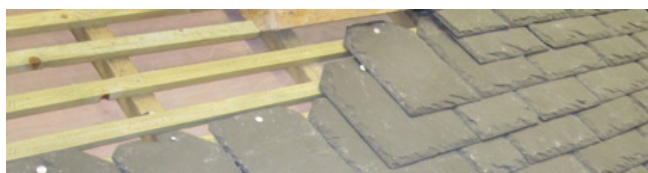
A modern roof using peg tiles
