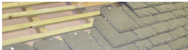
A modern roof using peg tiles
